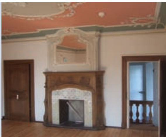
Right and top: Grafschafter Castle in the town of Moers, Germany is now protected by a high-pressure water-mist system.
